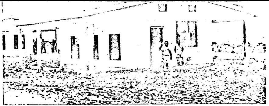
When 40 families, exiled to the island of Rongerik and later to Kili from their home on Bikini Atoll, return to their nuclear-bombed home, they will find these new houses waiting for them. Forty houses, built of concrete with iron roofs, toilet, laundry and cooking outbuildings and a large water-catchment tank, were scheduled for occupation by Christmas. Representatives of the Bikini people approved the design and inspected the completed dwellings during a special visit in November.
